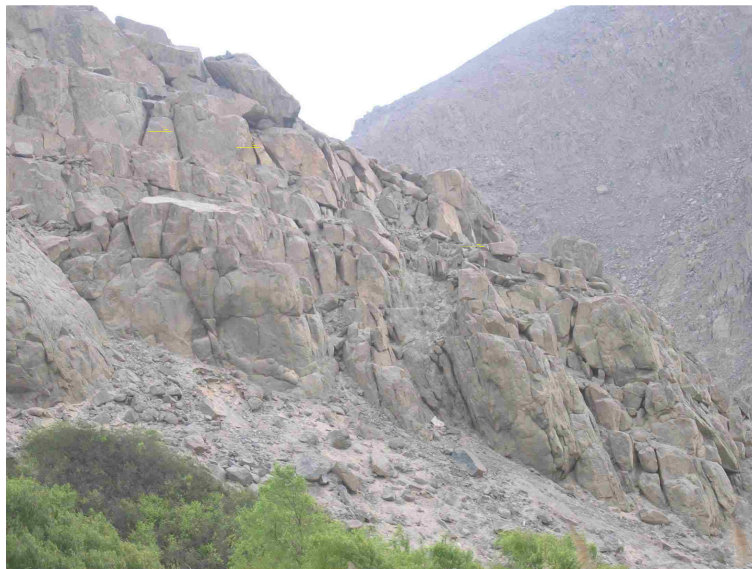
(b) Blocky slope with indications of rock blocks where sliding and slumping modes are suspected.
